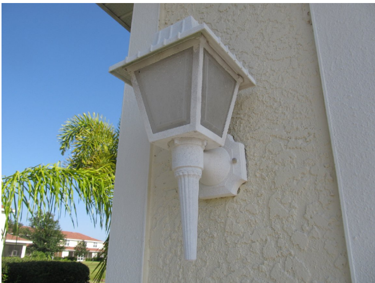
Light fixture at 1148-1158 Jonah Drive
