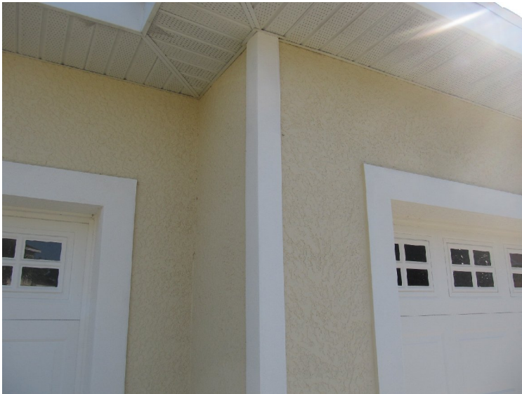
Exterior stucco finishes
