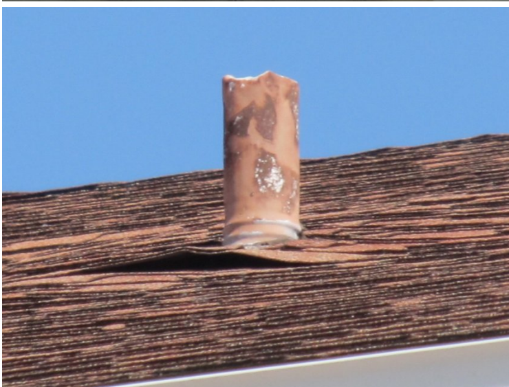
Asphalt shingle roof
