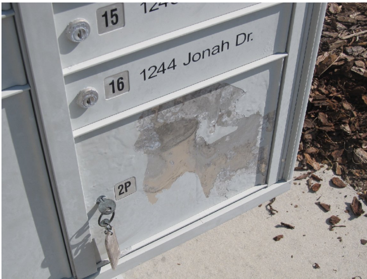
Isolated finish deterioration at mailbox station
