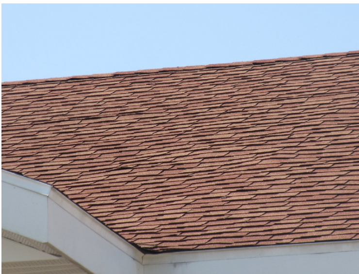
Asphalt shingle roof at 1149-1159 Jonah Drive
