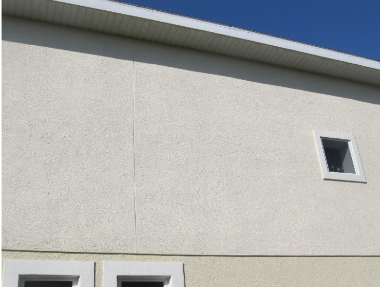
Exterior stucco finishes
