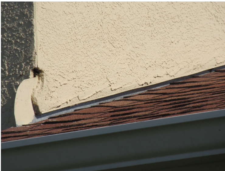
Asphalt shingle roof at 1088-1102 Jonah Drive
