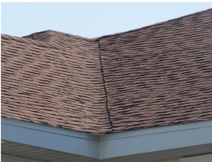
Asphalt shingle roof at 1329-1339 Rosewood Lane
