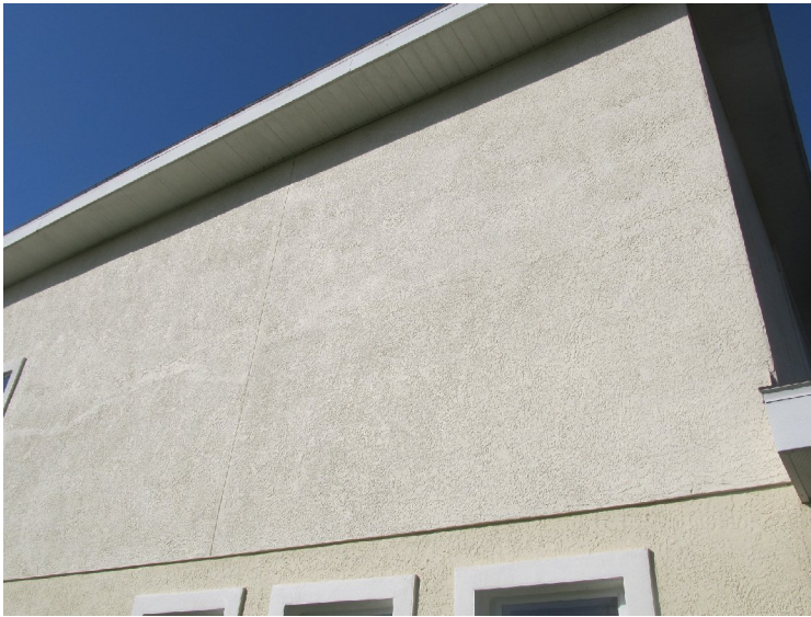
Exterior stucco finishes
