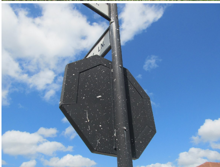
Stains at street sign
