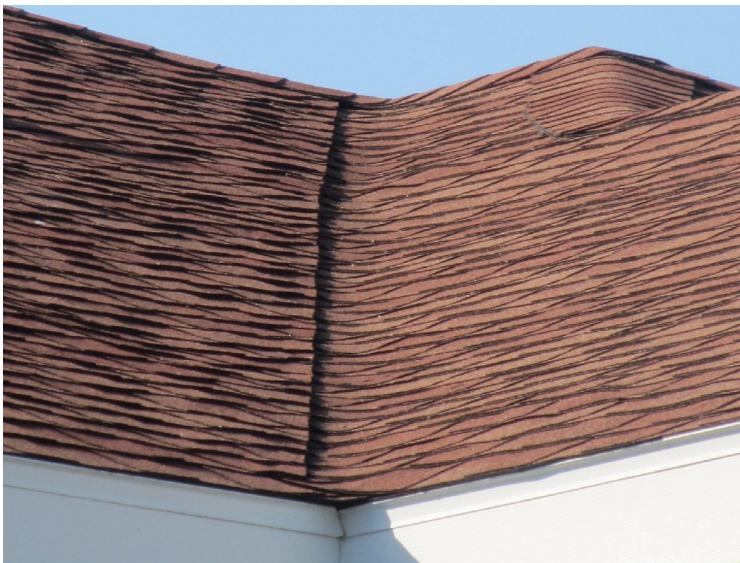
Asphalt shingle roof at 1050-1060 Jonah Drive
