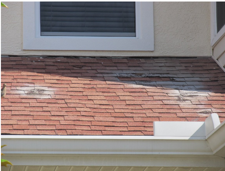
Asphalt shingle roof at 2346-2347 Felicity Way
