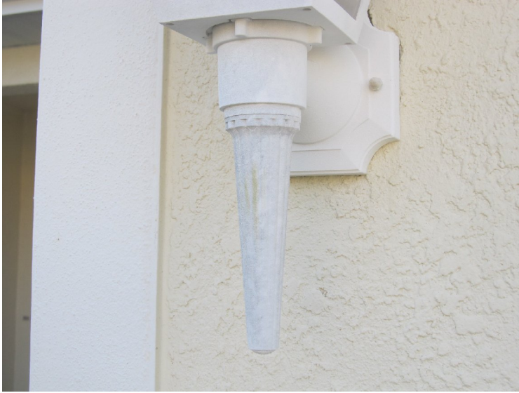
Light fixture at 1050-1060 Jonah Drive
