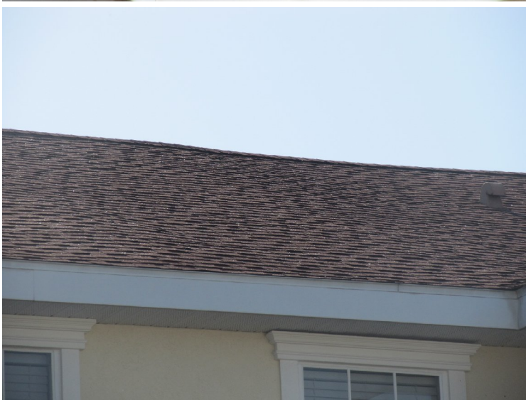
Asphalt shingle roof at 1088-1102 Jonah Drive
