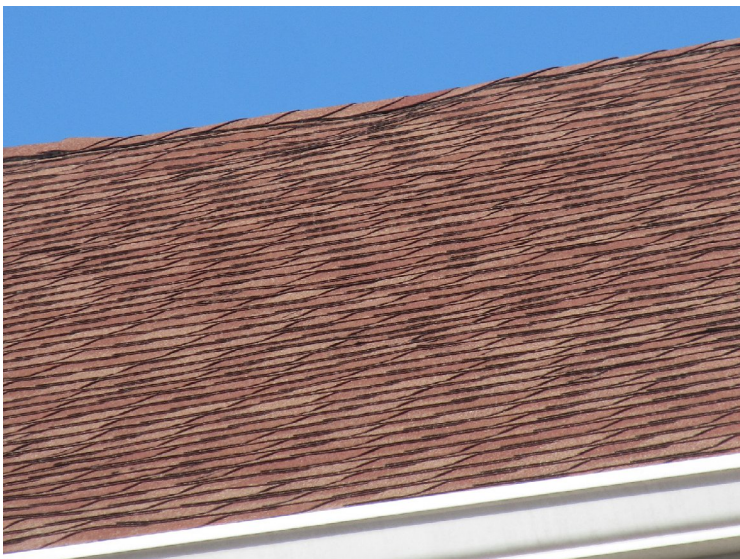
Asphalt shingle roof at 2265-2274 Mulberry Lane
