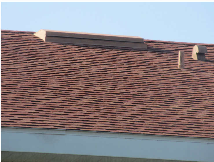
Asphalt shingle roof at 1057-1067 Jonah Drive
