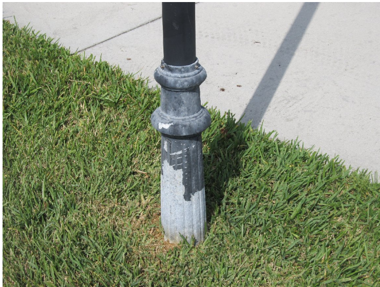
Finish deterioration at base of street sign
