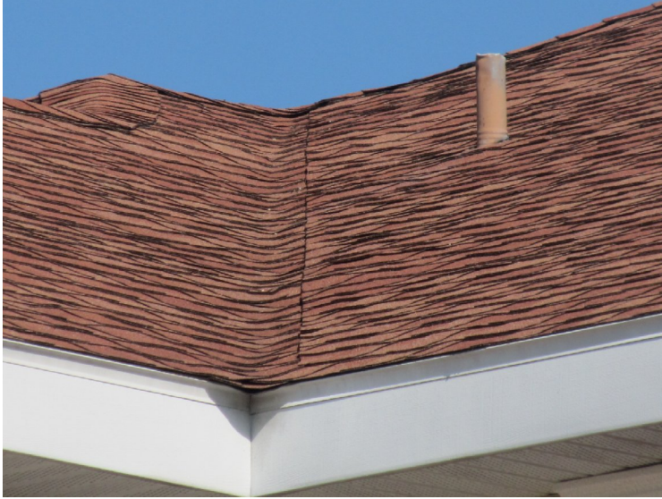
Asphalt shingle roof at 2349-2359 Rosewood Lane
