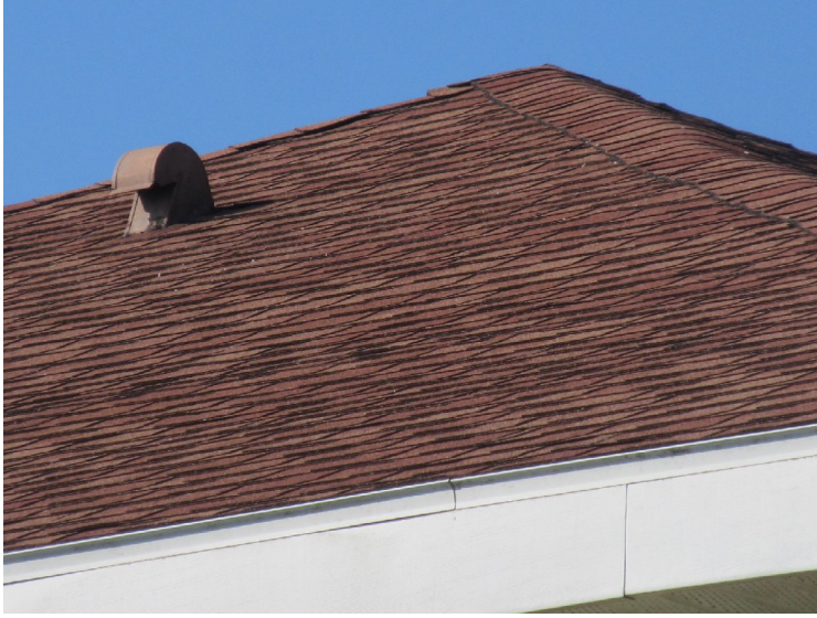
Asphalt shingle roof at 1071-1081 Jonah Drive
