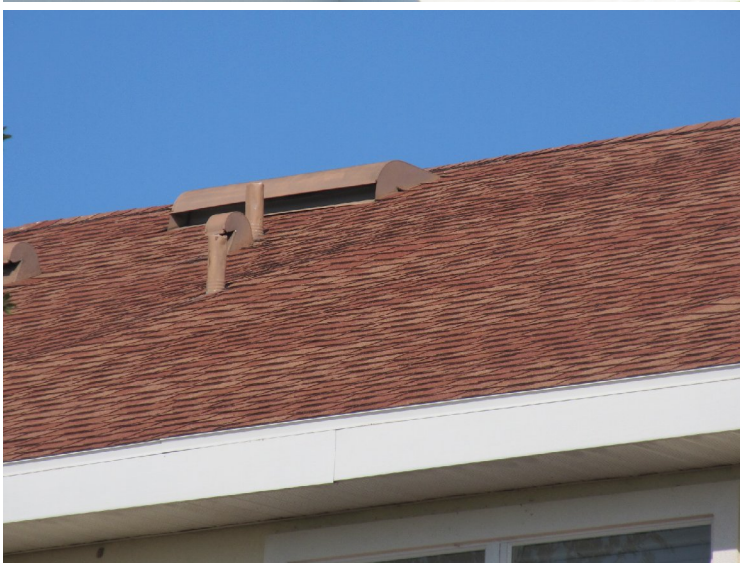
Asphalt shingle roof at 1064-1076 Jonah Drive
