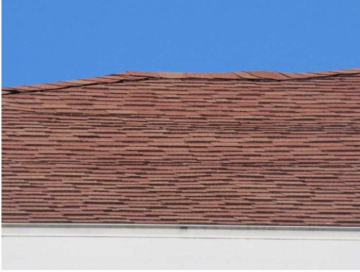
Asphalt shingle roof at 1057-1067 Jonah Drive
