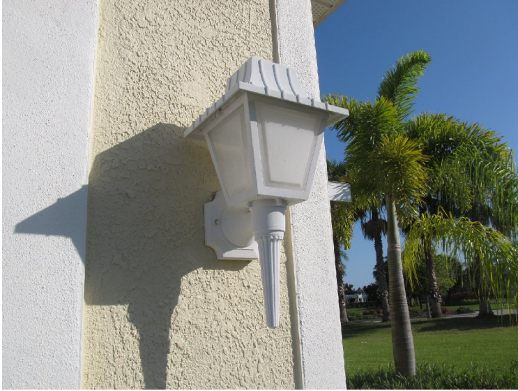
Light fixture at 1057-1067 Jonah Drive
