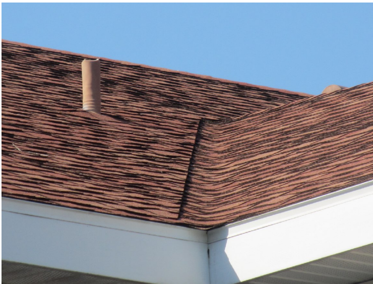
Asphalt shingle roof at 1129-2292 Mulberry Lane
