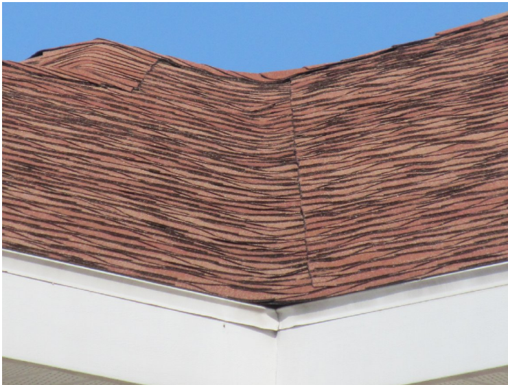
Asphalt shingle roof at 1057-1067 Jonah Drive
