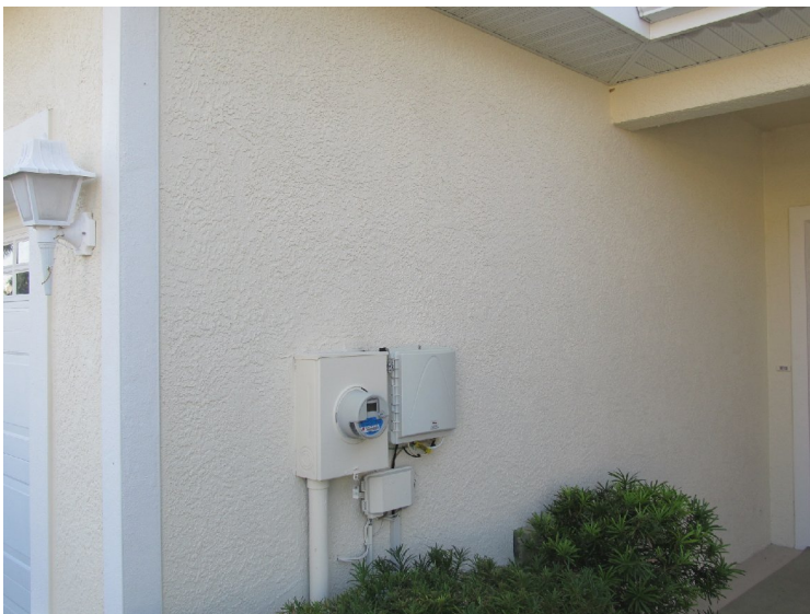
Exterior stucco finishes
