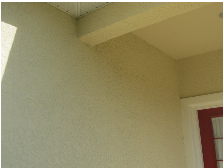
Exterior stucco finishes
