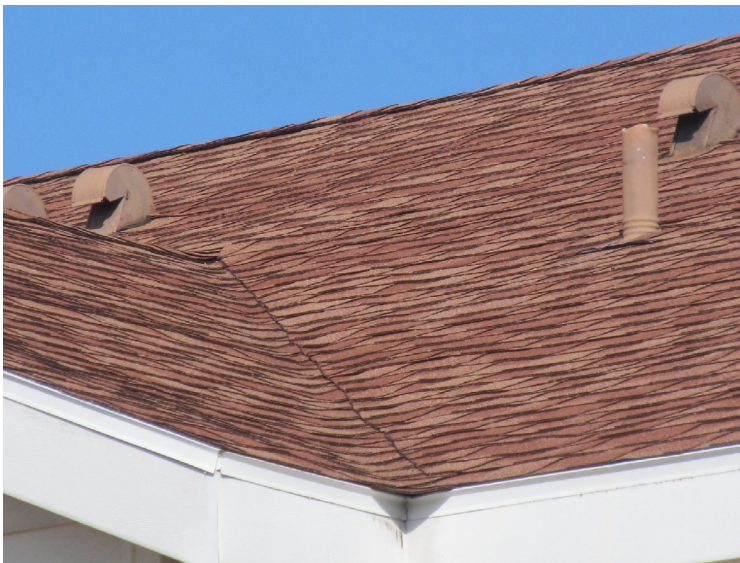
Asphalt shingle roof at 1071-1081 Jonah Drive
