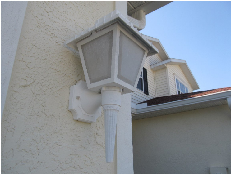
Light fixture at 1329-1339 Jonah Drive
