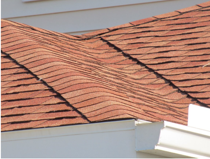
Asphalt shingle roof at 1128-1138 Jonah Drive
