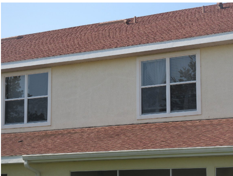
Asphalt shingle roof at 1128-1138 Jonah Drive
