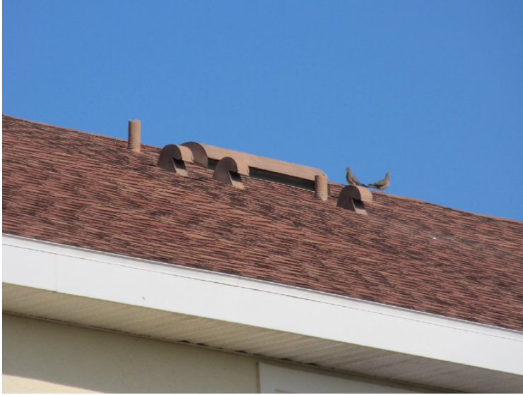
Asphalt shingle roof at 1088-1102 Jonah Drive
