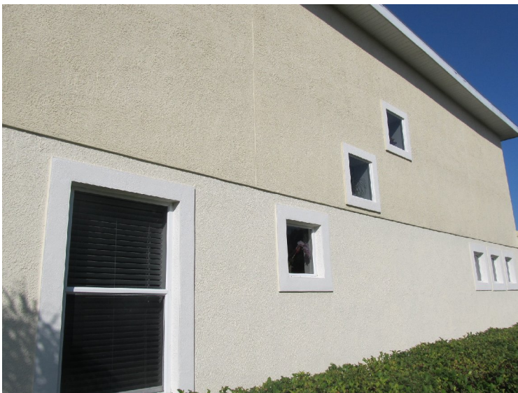
Exterior stucco finishes
