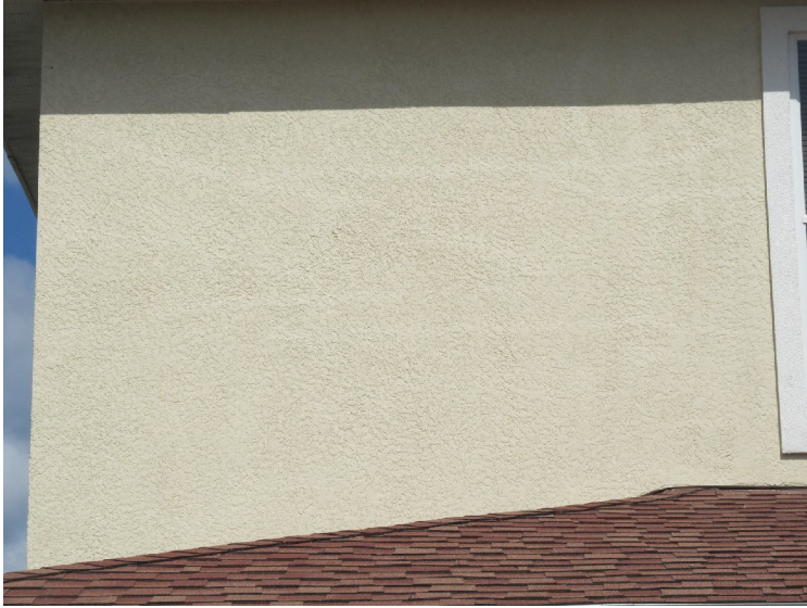
Exterior stucco finishes
