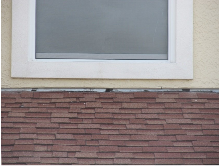
Asphalt shingle roof at 1214-1220 Jonah Drive
