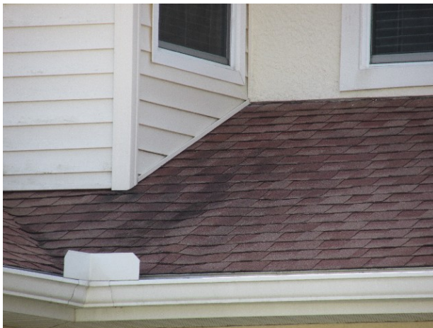
Deterioration and deflection evident
