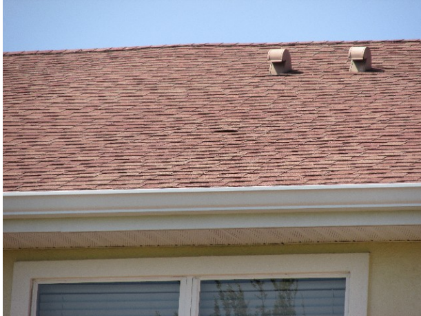
Shingle lift evident
