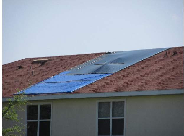
Roof leak under repair
