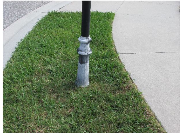
Finish deterioration
