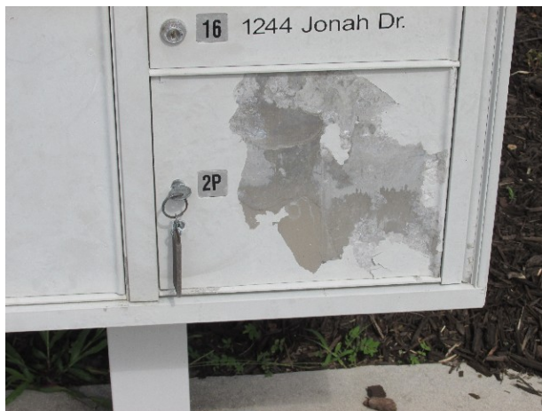
Finish deterioration evident
