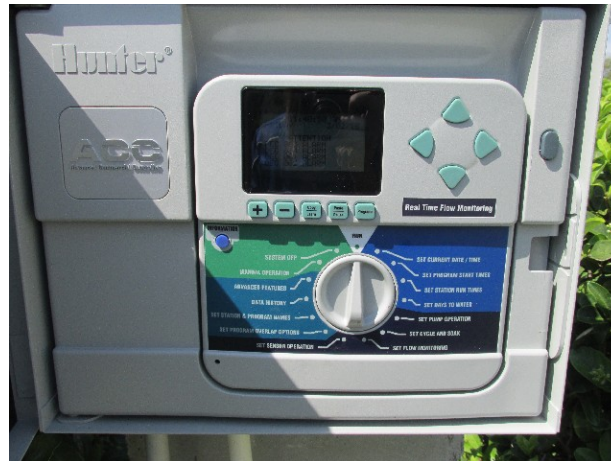
Irrigation controller
